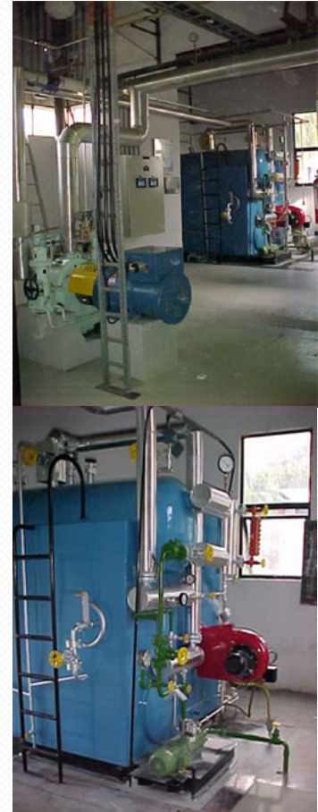
Figure 4 – 85 kw steam turbine with electric generator and aquotubular boiler by steam cycle
